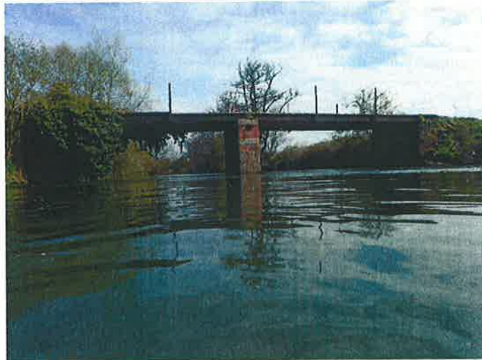
Black Bridge (BA37) Grid Ref: ST 90684 65027 South Elevation (Downstream)
